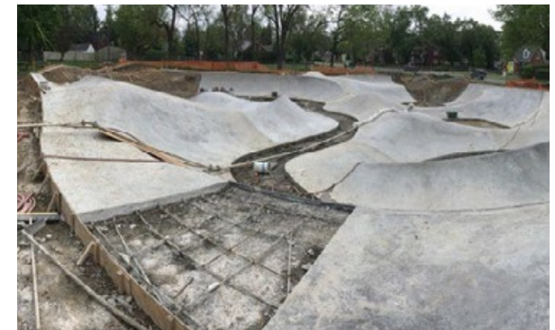
Skatepark Installation at Geary Park
