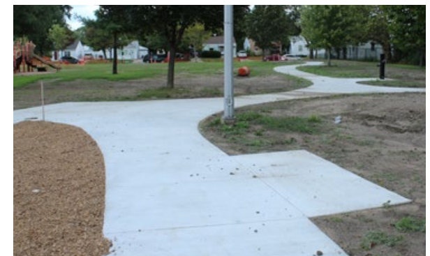
ADA walking paths installed at Wanda Park
