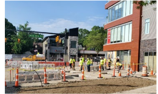
Schiffer Park under construction
